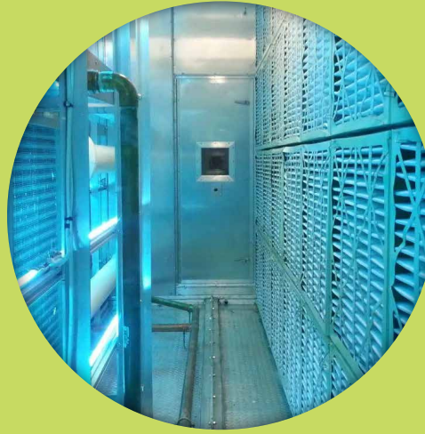
Induction of MERV 13 Filters & UVGI. to AHU's
